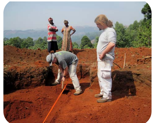
Mentors Dave Sacco and Jeremy Smith excavate and create a gradient in the site of the secondary storage tank
